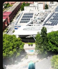
05 Def. Terrena · Drone and motion
